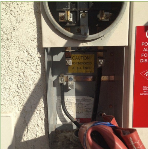
Exhibit #2 Completed Meter + GMA installation + wiring
